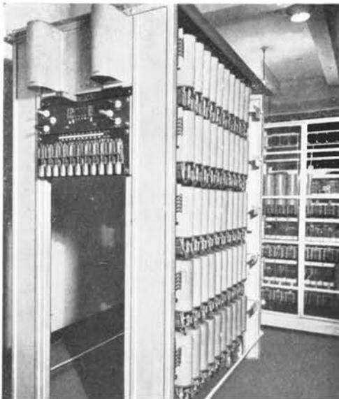
*Fig. 4—Dial-type private branch exchanges have usually been made in the larger sizes as indicated by this section of a 700 type*
