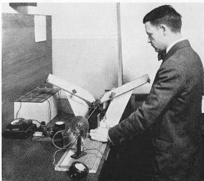
Experimental circuits for 60 cm. radio waves take some unusual forms. Four tuned circuits are present in this detector circuit being tested by J. G. Chaffee of the Research Department.
