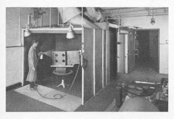
Fig. 2—Mounted on a turntable in the large power-ventilated spray booth, big apparatus is sprayed by Thomas Cassidy. The apparatus is later dried in the oven directly behind the booth
