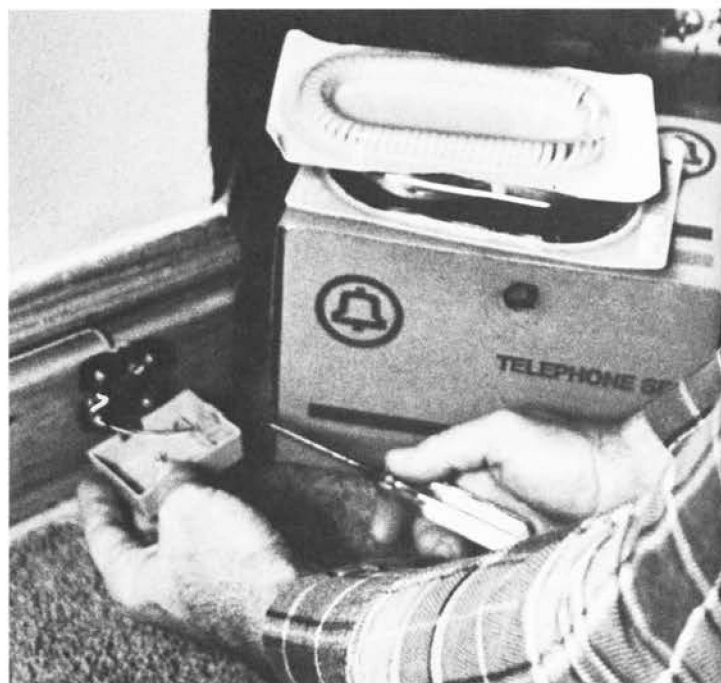
Converting an existing installation is simple. A new cover containing an integral modular jack fits over the standard terminal block. Here the spade-tipped jack leads are attached to the customer's wall terminal block before the new cover is put in place.
