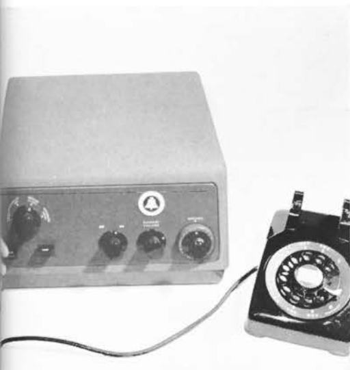
The 1-type answering set, developed by the Bell Telephone Laboratories.
