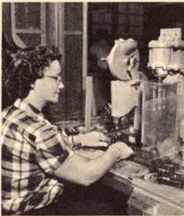
This member of the network assembly group in the Indianapolis plant performs two operations: she rivets the capacitor bracket and clinches the induction coil to the terminal plate. Over 60 Indianapolis employees work in the network assembly group.
