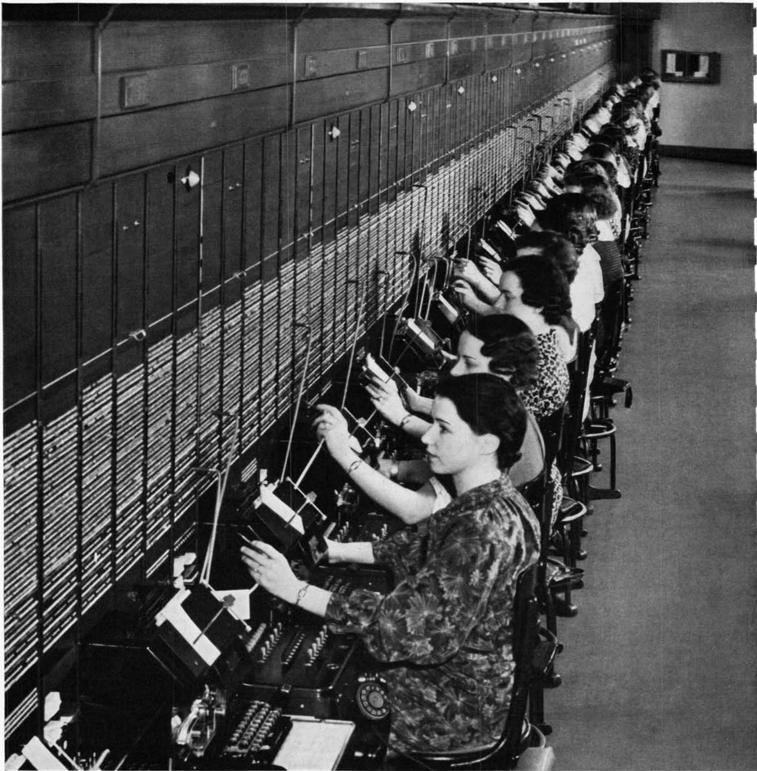
**Teletypewriter exchange service** — Teletypewriter exchange service is furnished on substantially the same basis as telephone service except that communication is typewritten instead of oral. Teletypewriter stations are connected to central offices, similar to the one pictured here, and through these central offices communication may be established with other teletypewriter stations similarly connected in the same city or in any other city.
