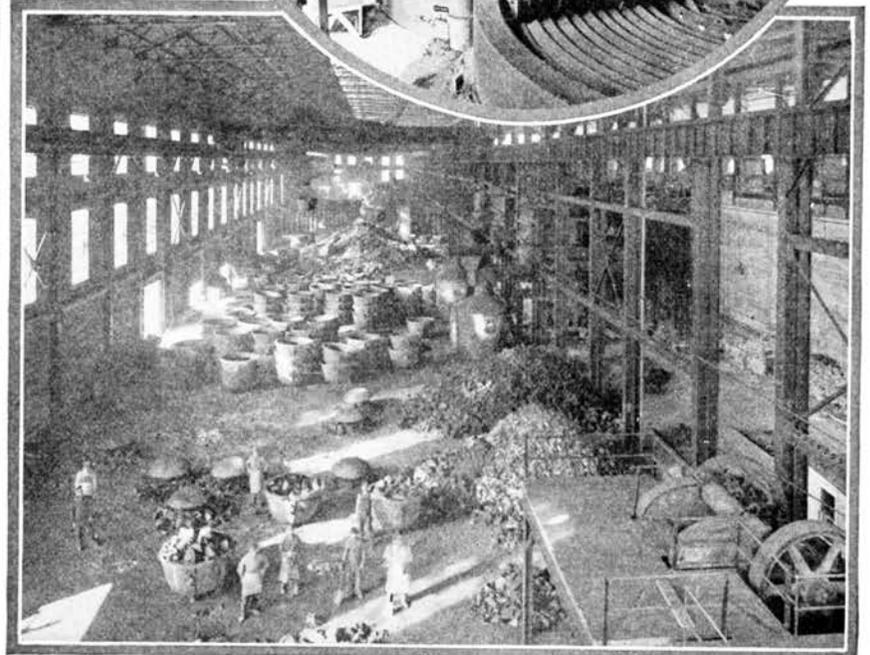
*Part of the operation of scouring nickel from its ore is done in cupolas such as these.*
