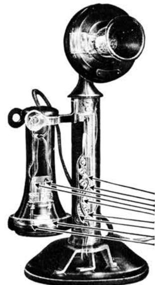
*Tin is a part of the solder which makes firm good current carrying connections between many of the small parts in your telephone.*
