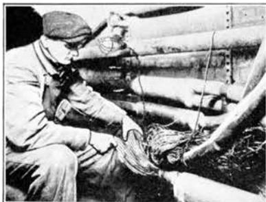
*Solder joins the wires in lead covered cables and also joins the lead sheaths where two cables come together, thus preventing moisture from creeping in to injure the insulation.*
