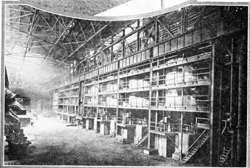
*The zinc oxide falls through these bags to bins from whence it is barrelled while the gases pass out through the pores of the bags.*
