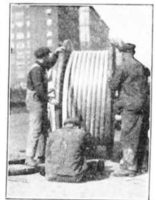
In this familiar scene the telephone wires are being put underground enclosed in their protective sheath of lead and antimony.
