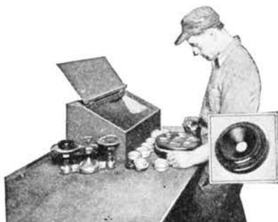
*Rubber dust is poured into moulds like that the operator has before him and dies are inserted. When heat and pressure have vulcanized the rubber contents of the mould, receiver caps result, ready to be smoothed to the glass-like surface you have so often felt against your ear.*
