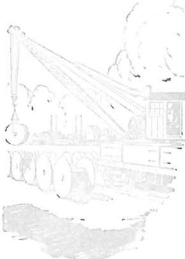
This electric storage battery crane locomotive handles cable reels and does the work of many men.
