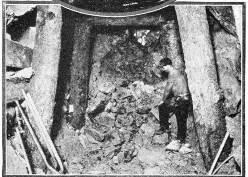
*After the blast, the broken rock is taken away, broken into still smaller pieces and processed to obtain the various metals it may contain. The "timbering" is to keep the roof and walls from caving in.*
