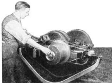
*For telephone work platinum frequently must be drawn into wire, some of which is later rolled into thin ribbons and some is used as wire in the switchboard lamps and vacuum tubes*
