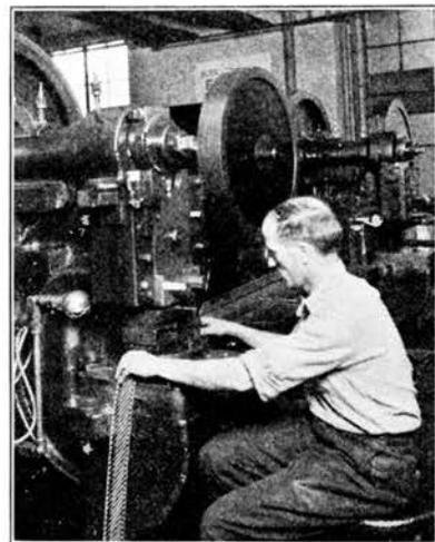
*Tens of thousands of springs containing nickel are used in making telephone equipment. To make sure each is exactly like all the others for the same purpose machines like this punch them out of long strips of metal.*
