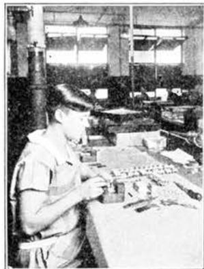
*Thin sheets of mica are assembled for the condenser which controls the flow of current and gives the greatest possible clearness to words.*
