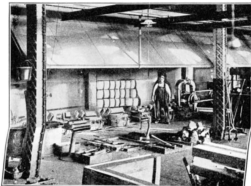
*In this brass foundry immense quantities of zinc are alloyed with other metals to make the thousand and one brass parts used in telephone switchboards and elsewhere in telephone apparatus.*
