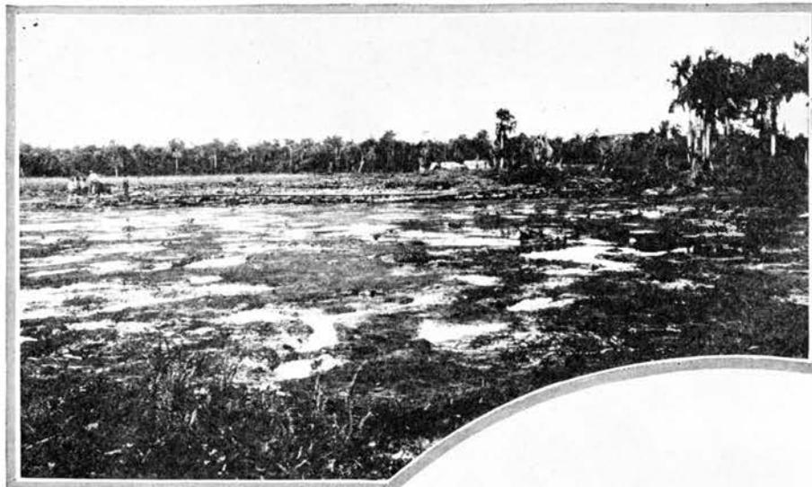
*Below—The Trinidad Lake of Asphalt is very different in appearance from the Bermudez Lake. It is practically an uninterrupted sheet of asphalt. Here, too, light railroads that are moved as the surface of the lake moves, transport the asphalt.*
