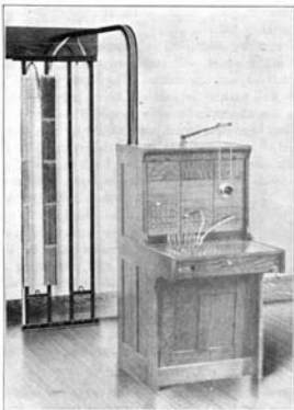
Fig. 26—Two No. 1 Protector Frames and No. 1 Cable Rack installed with No. 105 Switchboard
