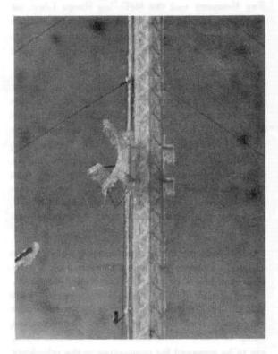
About half of the antenna systems on short haul routes in the Bell System utilize reflectors. A recent survey shows that prior to this Michigan case the system has experienced over 1300 reflector years of service since 1951 with six cases where falling ice damaged the dishes below. Three of these cases resulted in a few hours of service outage. This experience has been good; however, the possibility of falling ice should not be overlooked.
