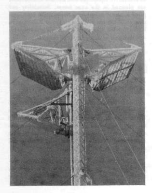
tures withstood the ice load; however, falling ice damaged the dish antennas directly below causing a twenty-five hour service interruption.
