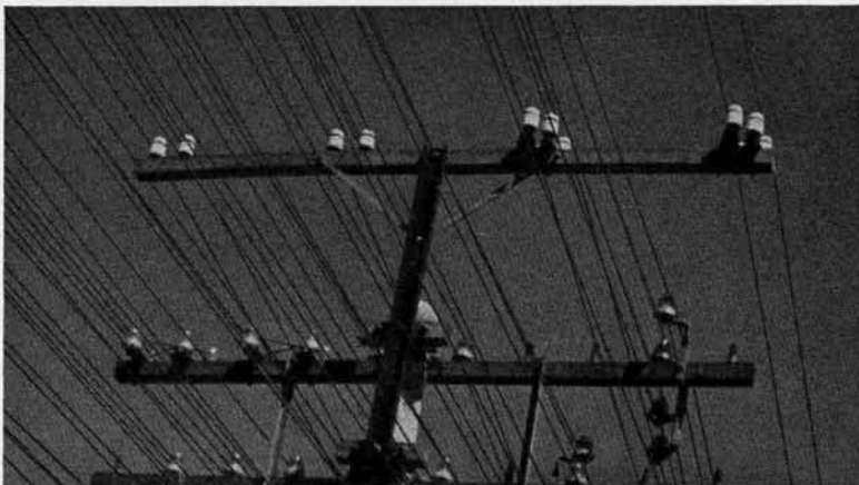
Figure 12—Typical crossarms, insulators, and transposition brackets. The zero crossarm carries 5.9-inch (15-centimeter) spaced wires on type-2 porcelain insulators mounted on H-15 -type transposition brackets. The first crossarm supports wires with 11.8-inch (30-centimeter) spacings; they are carried on double-petticoat alkaline-glass insulators mounted on both point- and drop-type transposition brackets.
