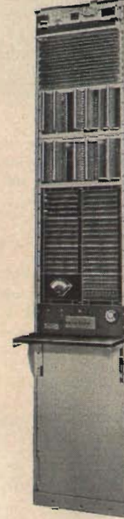
● Outgoing trunk test bay.
