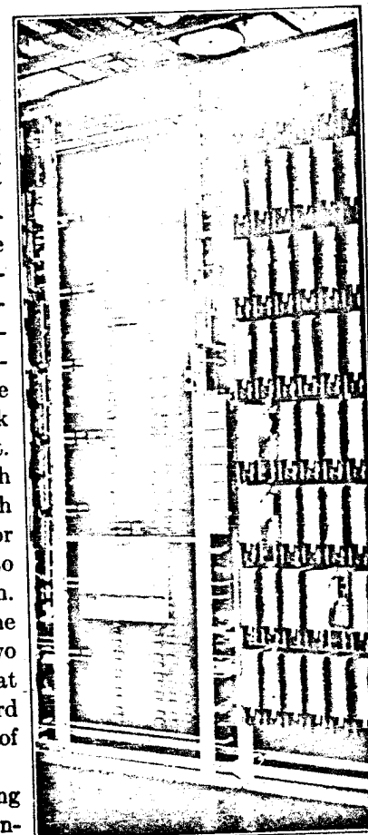
FIG. 85.—Selector distributing terminal assembly frame.
