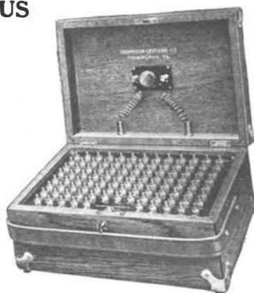
100 Cell Silver Chloride Testing Battery
