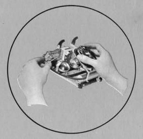
It's a simple matter to add a dial, in case your exchange is converted from magneto to dial service. The dial mounting bracket slips in place and the dial cords are attached to the convenient connector block.
