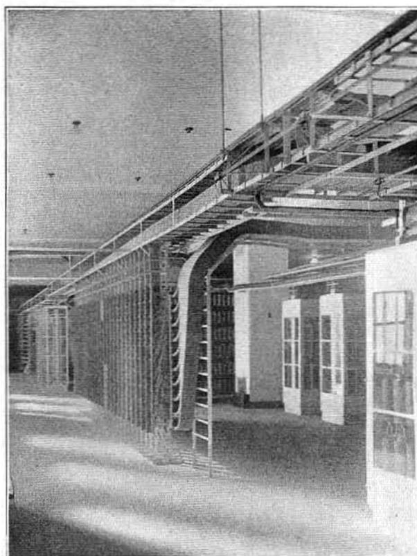
Fig. 66. View of switchroom showing intermediate distributing frame
