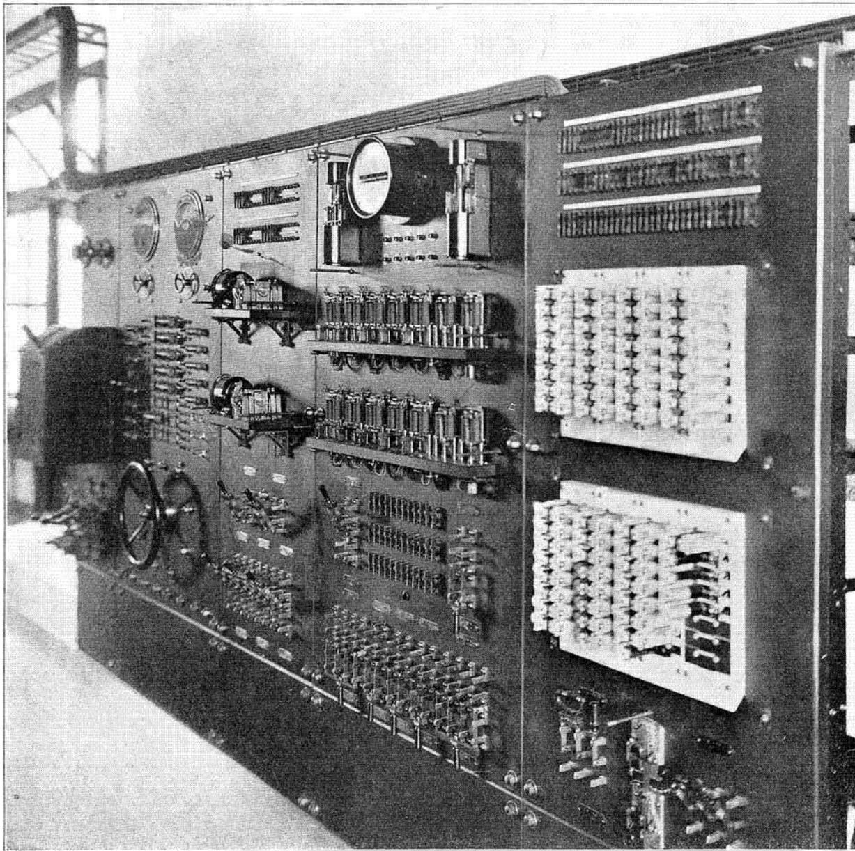
Fig. 56. Typical power board for automatic exchange
