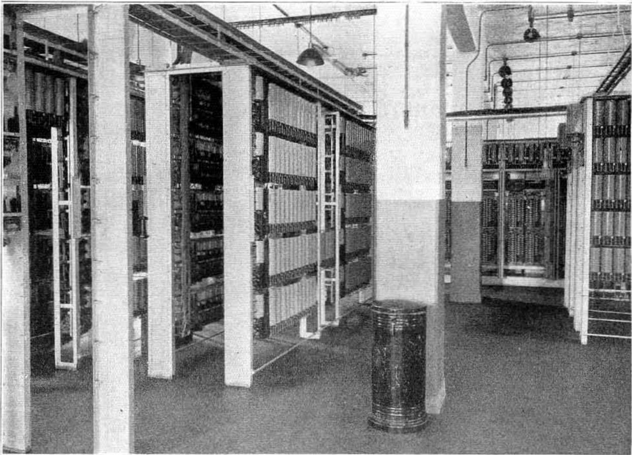
Fig. 48. Switchroom view, showing connectors and secondary line switches installed
