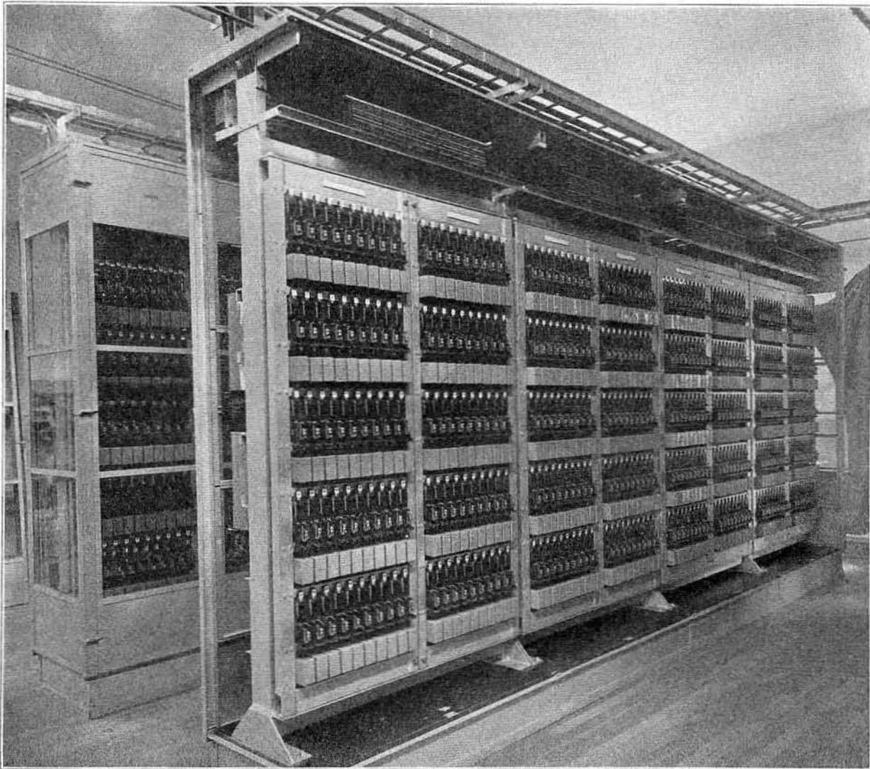
Fig. 47. Switchroom view, showing rotary line switches installed
