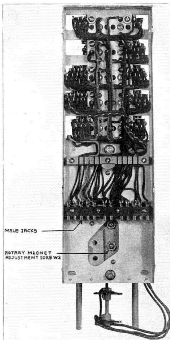
Fig. 11. Rear view of connector showing wiring
