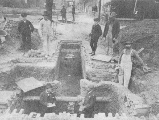
Constructing the Lincoln office manhole in the autumn of 1903. The gas main seen in the picture still bisects our present office manhole.
