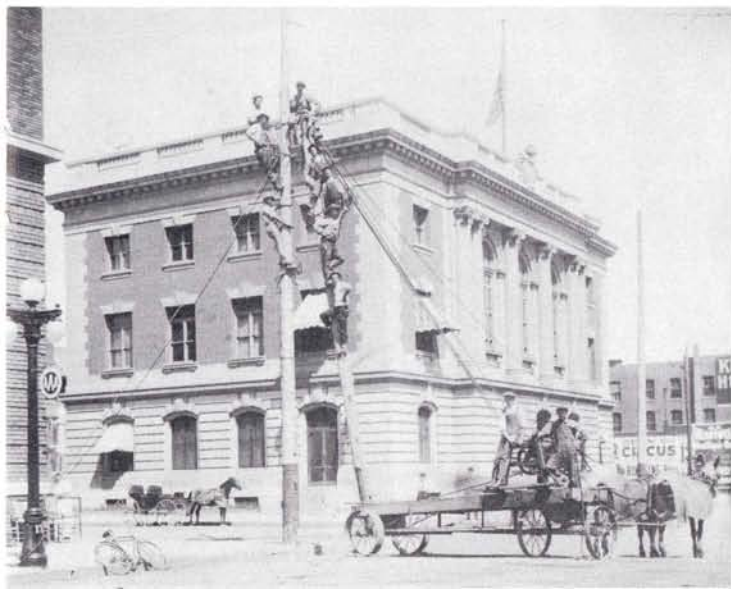
The "pole gin" in use at Hastings rebuild in 1914. J. L. Lyne, present outside plant engineer, is the youngster in overalls and light shirt standing at left on truck bed.
