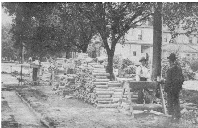
Laying underground conduit south from the office in 1903. Residences in background occupy site of present general office building.
