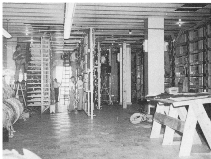
By late August 1952, the second floor was occupied by rows of switching equipment, with the Automatic Electric installation crew busily engaged in making the multitudinous and necessary connections.
