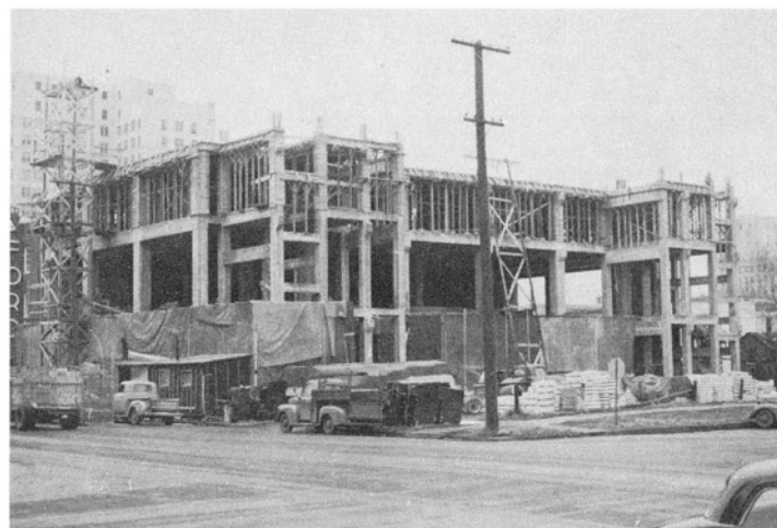
During the winter of 1951-52 the first floor was enclosed with tarpaulins while masons and construction crews continued their labors on the interior. Most of the pipe runs and busducts were completed by mid-March, 1952.
