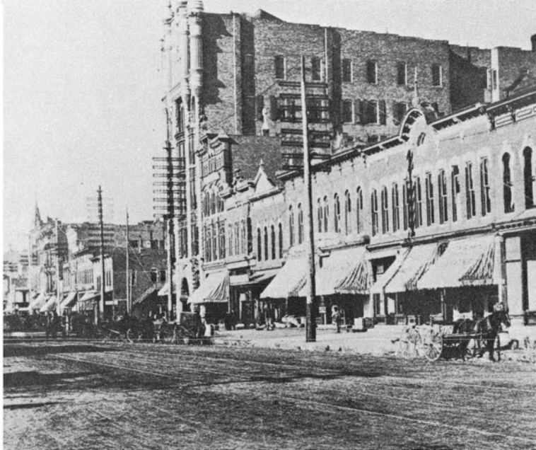
Lincoln was a flourishing city at the turn of the century but even the downtown subscribers were connected by aerial wire leads supported by self bracing double arms. This is O Street, looking west from 13th.
