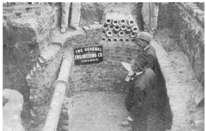
Another view of the office manhole, 1903, showing the entrance of concrete ducts from the north. The men are engineers for the contractor.
