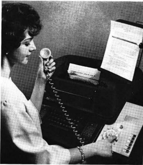
An attendant uses the new subscriber set on a teletypewriter console equipped for dial TWX service.
