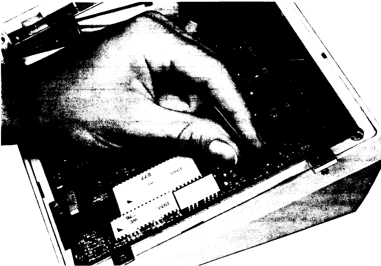
Fig. 5—2870A1 Dial, Connection of D-180818 Kit of Parts, Record Disable Feature Only
