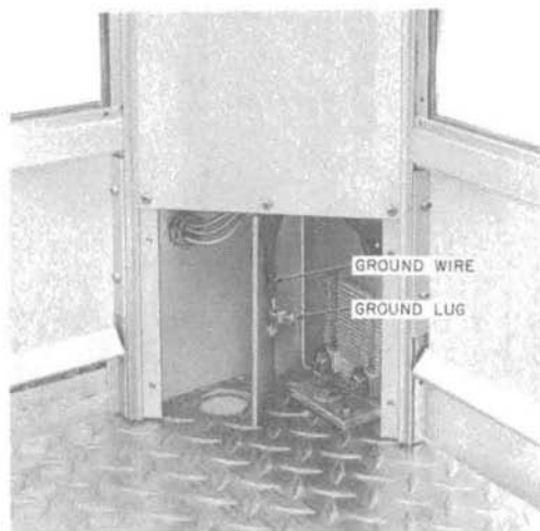
Fig. 6—Grounding Screw in KS-19580 Booth
