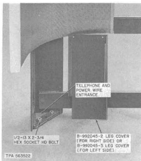
Fig. 22—List 14 Leg Assembly Bolted to Mounting Surface
