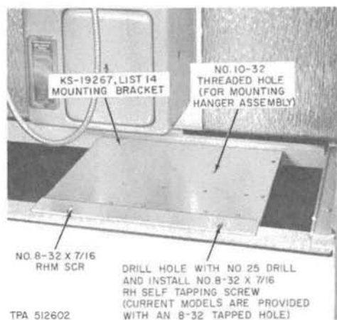
Fig. 15—Locating KS-19267, List 14 Mounting Bracket
