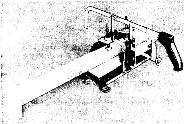
**Fig. 3—Waveguide Section Clamped in Position with Hacksaw Assembled**
