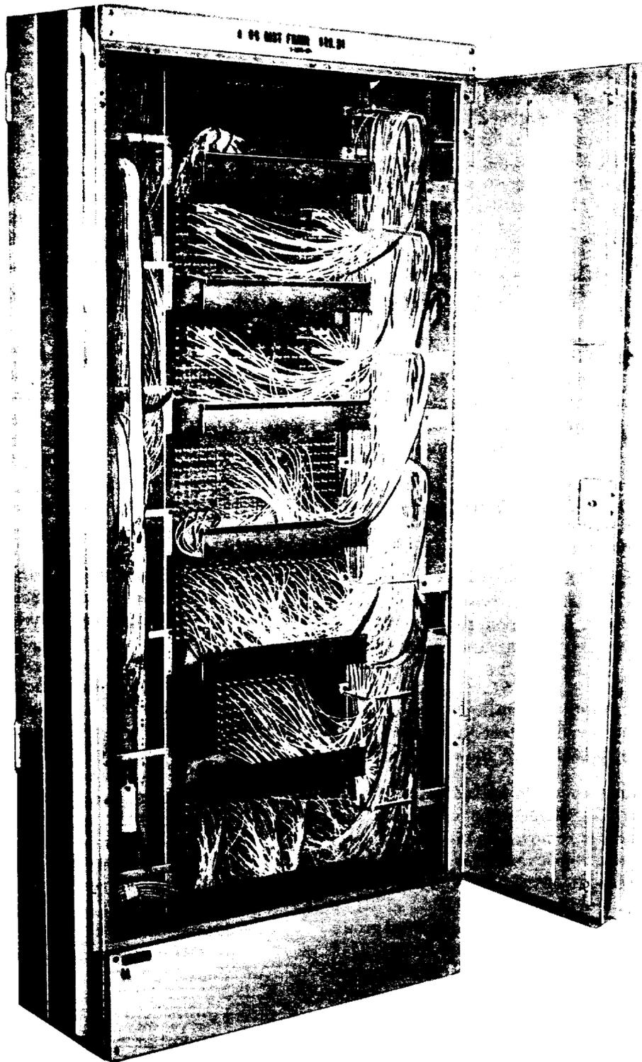
Fig. 5—Type I Supergroup Distribution Frame Installed in Cabinet
