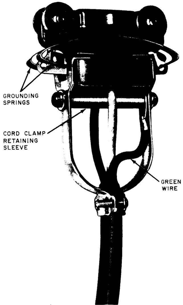
Fig. 7—KS-20085 L12 Terminal Trolley
