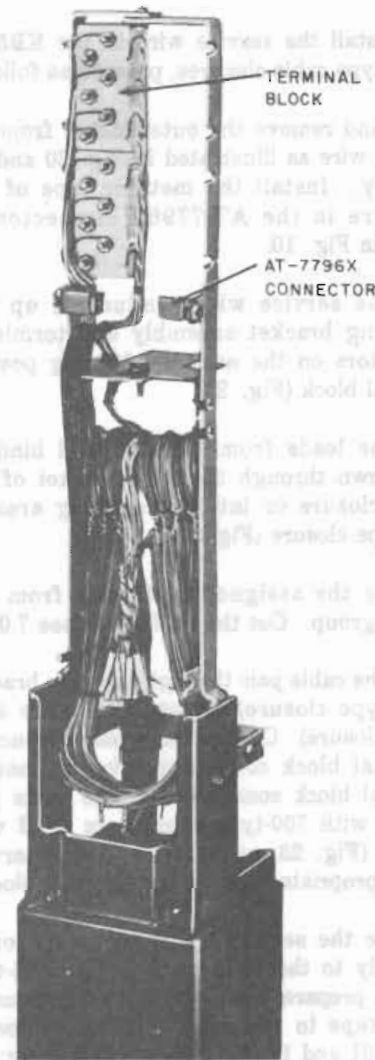
KC5 CABLE CLOSURE WITH TERMINAL BLOCK
