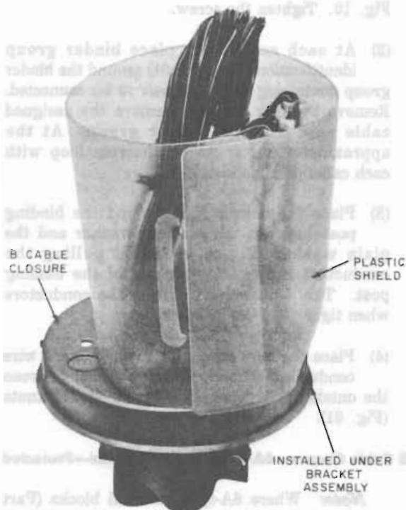
Fig. 63—B Closure Shield Installed in B Cable Closure
