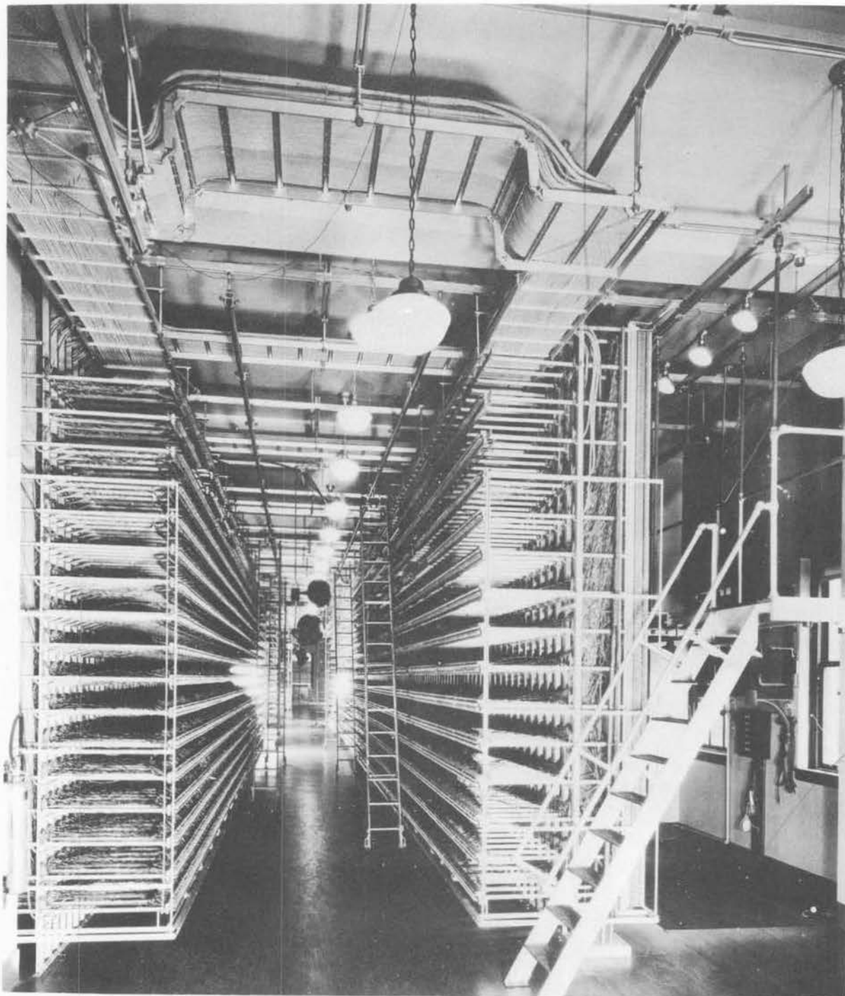
Figure 31 - Main and Intermediate Distributing Frame
