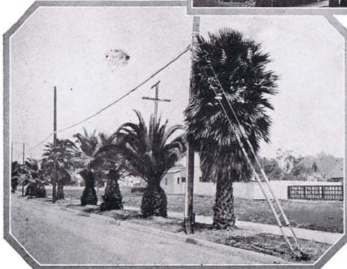
Underground pole and 600 pair aerial cable
