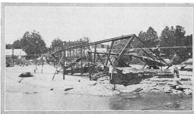
Above bridge after being razed. A span swung in the wrong direction and fell against the cable.
